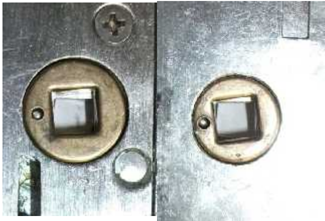
LH Side Fullex (New) RH Side Ball Bearing insert
