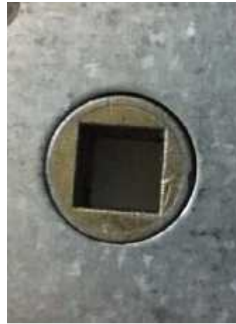
LH Side Maco (Old) RH Side Distinctive outer ring around circumference of spindle
